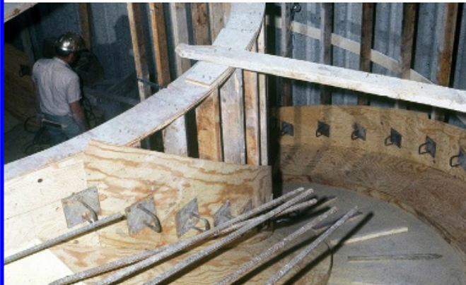
Constructing the Main Stairway
