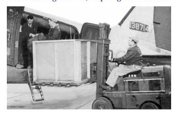
The most noticeable exterior difference between the "SkyTrain" and the "standard" DC-3 / C-47 was this front-opening "barn-door" combined with a rear-opening "standard" door. The large "hole" required strengthening the fuselage structure and also "beefing-up" the floor to support the weight of a jeep (or two). "Cabin" differences included fold-up aluminum & canvas "bucket-seats".
