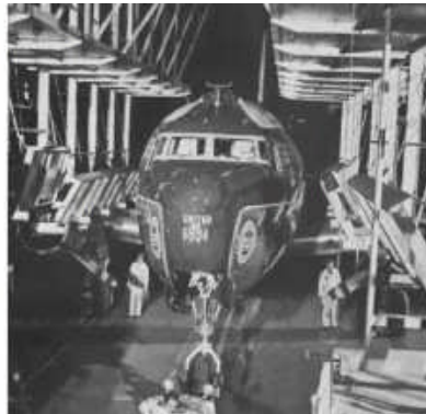
DC-6 in the hangar dock (center). The dock platforms on each side are lowered, allowing easy access to all the airplane's exterior surfaces.
